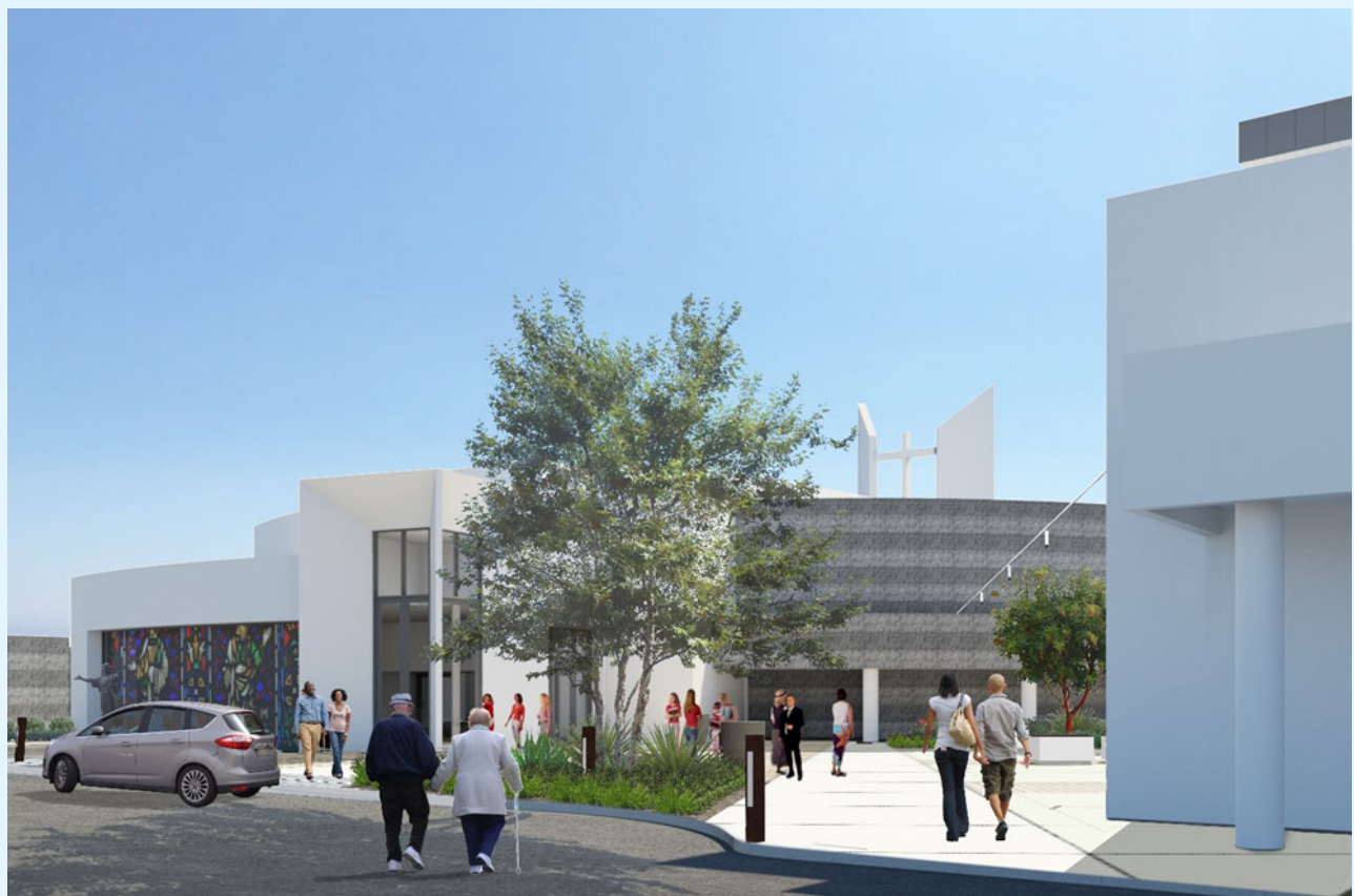
Figure 2: Narthex West View featuring new open entrance and exterior doors.
